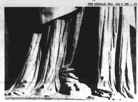
Miss Liberty's robes are made from finished sheets of copper, each just 3/32 of an inch thick and fastened to an internal skeleton
